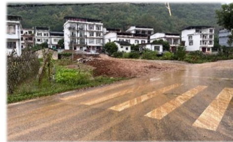
Bulks of Mud and Piles of Rubbish after the Flood
